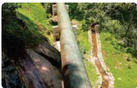
Surface vegetation and draining system to prevent soil erosion
